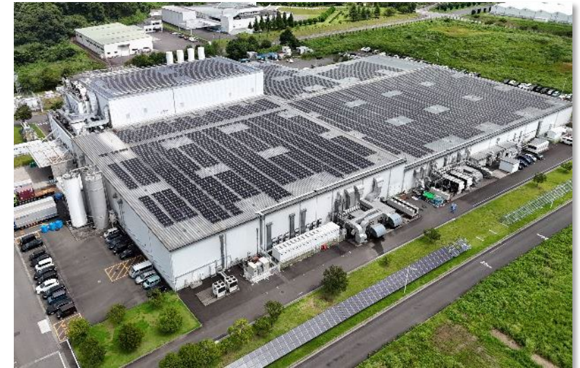
Solar power generation equipment at the Izumizaki Plant
