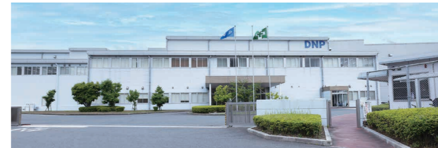
Exterior of the Kurosaki Plant in Fukuoka Prefecture
